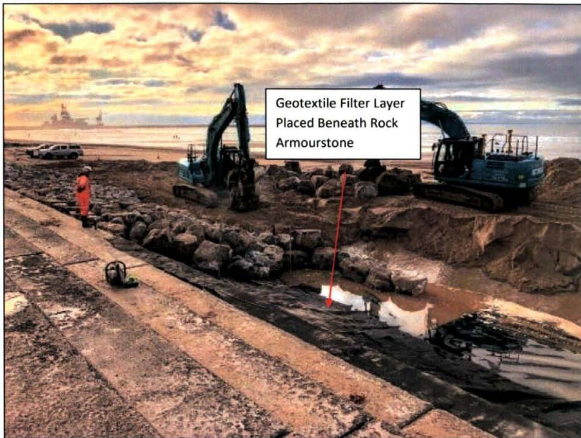
Figure 2.9 shows a typical arrangement of laying geotextile as a filter layer beneath the main rock armourstone in a coastal revetment.
