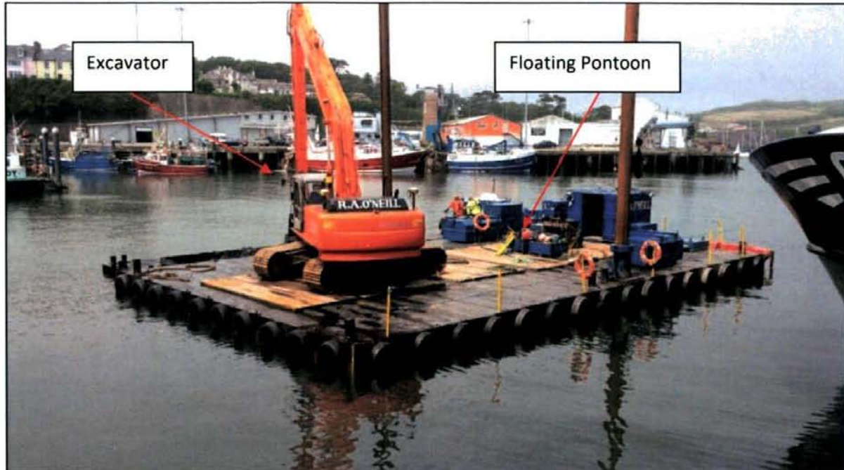
Figure 2.12 Example dredging operations using a floating barge and long reach excavator.
