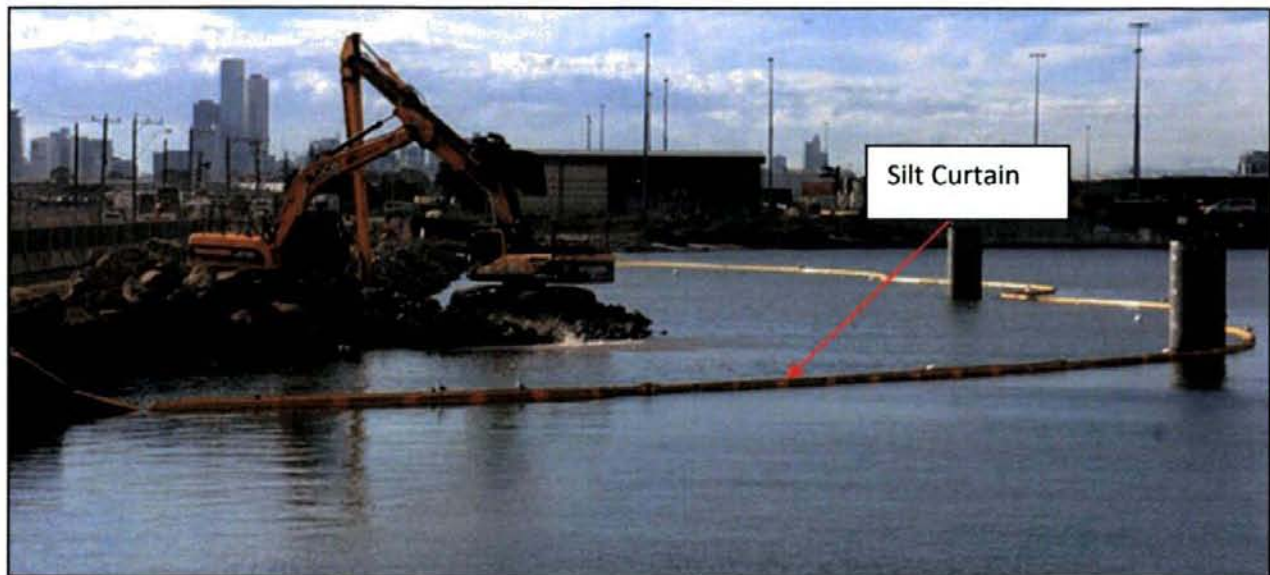
Figure 2.15 Example silt curtain arrangement surrounding dredging activities.
