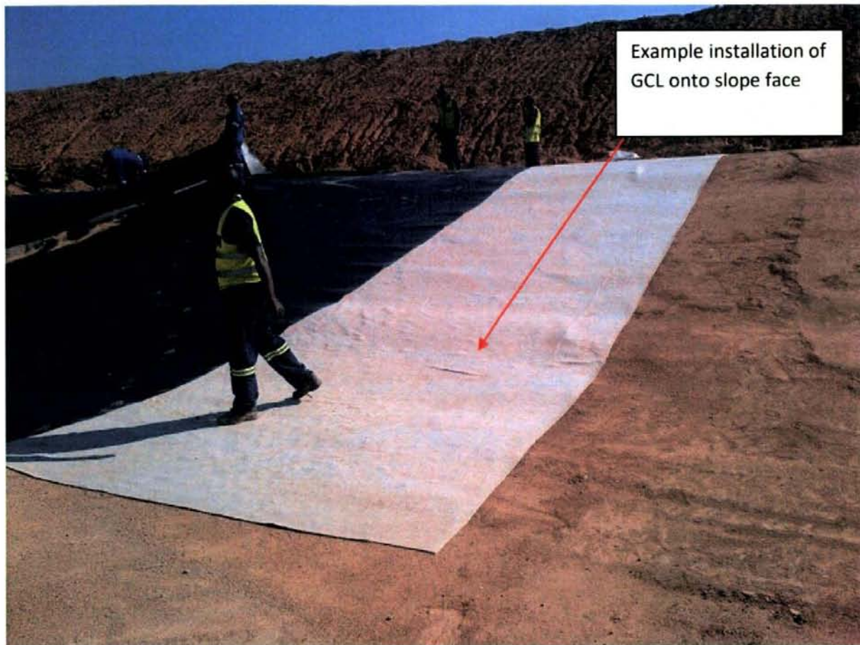
Figure 2.12 Showing a typical Geosynthetic Clay Liner (GCL) installation process.
